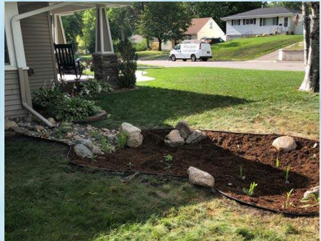
Raingarden capturing roof runoff
