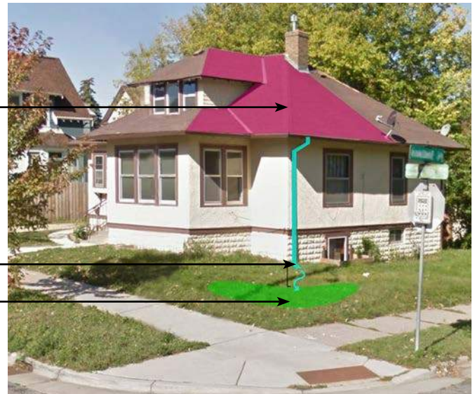
Raingarden capturing specific part of roof
