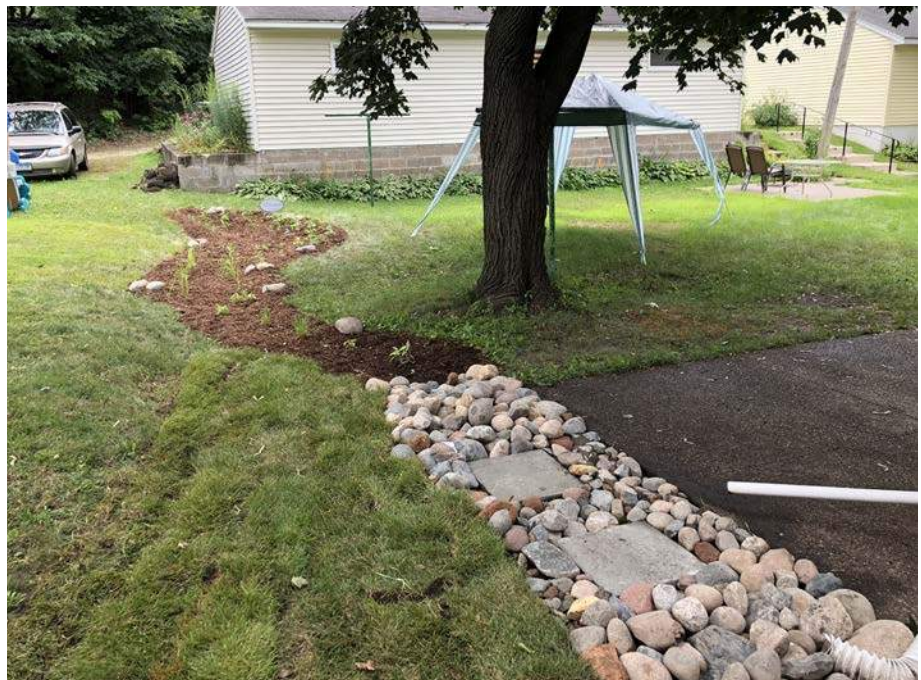
Downspout and sump pump to dry creek bed
