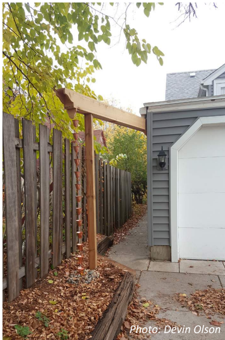
Overhead conveyance to rain chain
