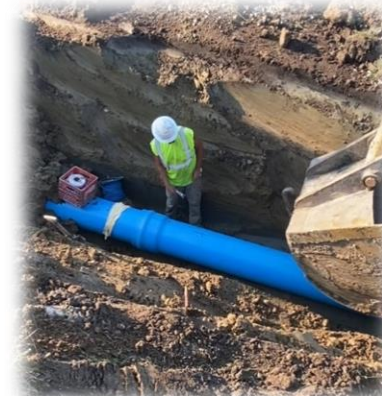
Watermain & Service Replacement
