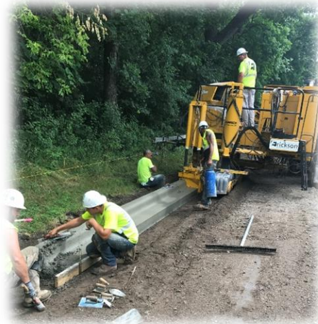
Concrete Curb & Gutter Installation
