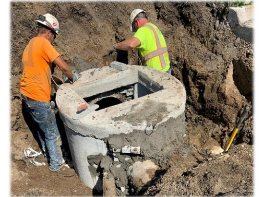
Storm Sewer Installation & Stormwater Management
