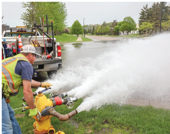
Water main flushing typically occurs each spring, which helps improve water quality by removing sediment.
