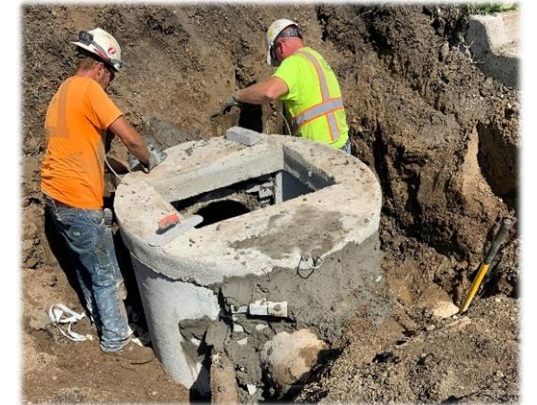
Storm Sewer Installation & Stormwater Management
