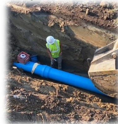
Watermain & Service Replacement
