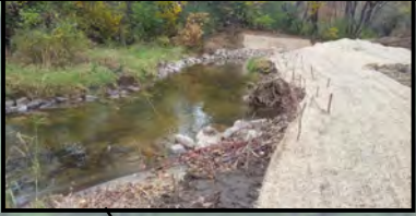
Example Rock Toe (Left) and Coir Blanket/Live Stakes (Right)
