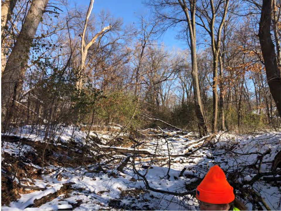
Figure 3-4 Debris and Left Bank Erosion (Reaches 1 and 2, downstream of upstream flared end section)
