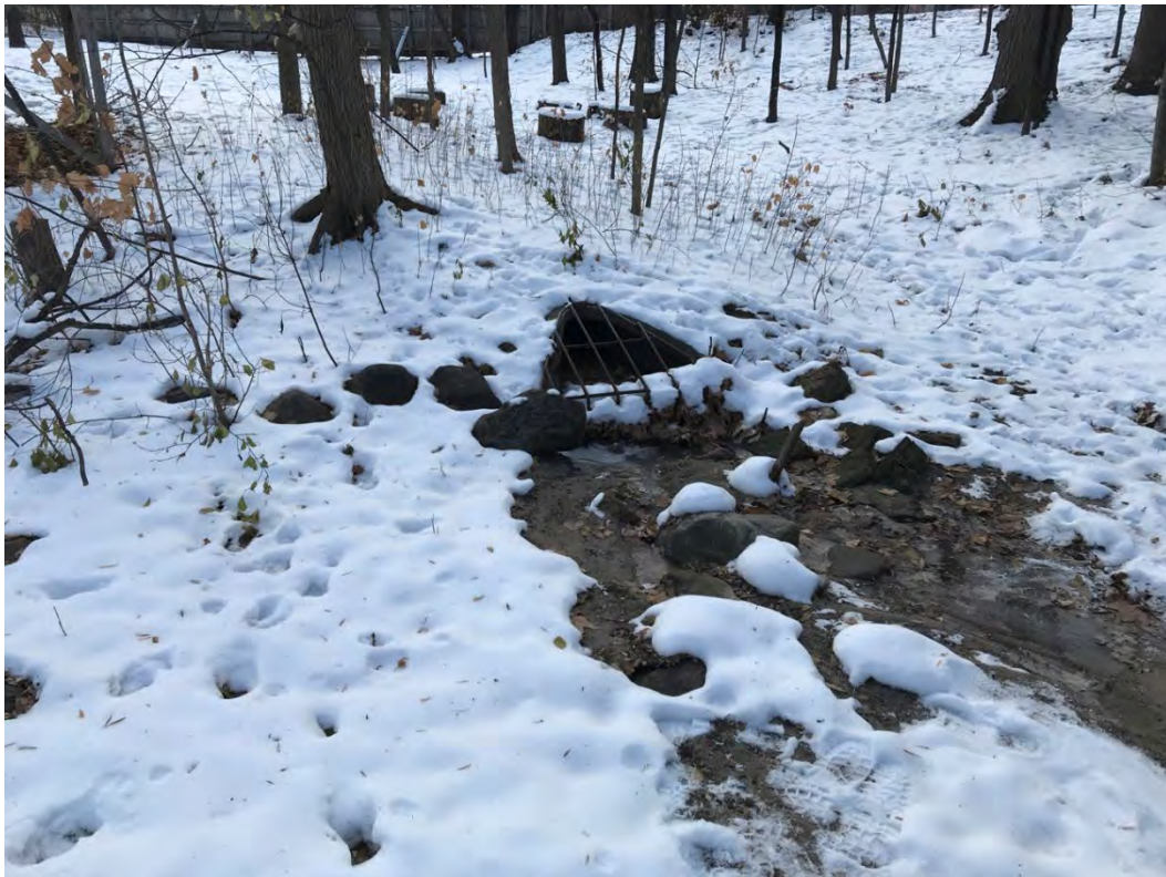
Figure A- 14 Upstream end of southwest stormwater side-channel.
