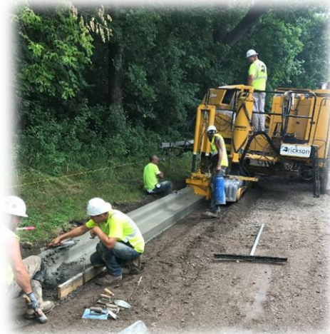
Concrete Curb & Gutter Installation
