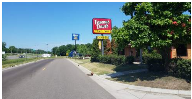
Lack of pedestrian facilities along the Frontage Road
