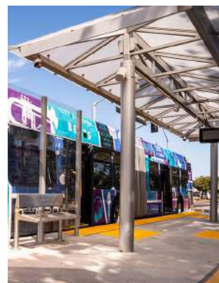
Transit station platforms
