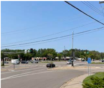
Highway 55/County Road 73 intersection
