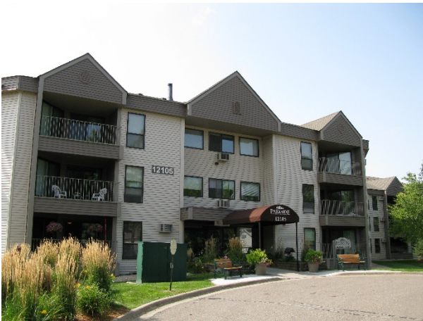
Parkside Apartments 12105 41 st Ave N
