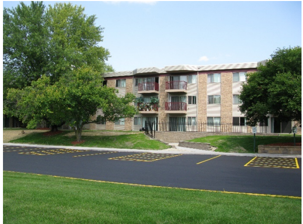
Manor Royal Apartments 3930 Lancaster Ln N
