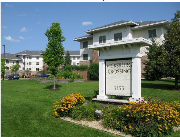
Vicksburg Crossing 3155 Vicksburg Ln N
