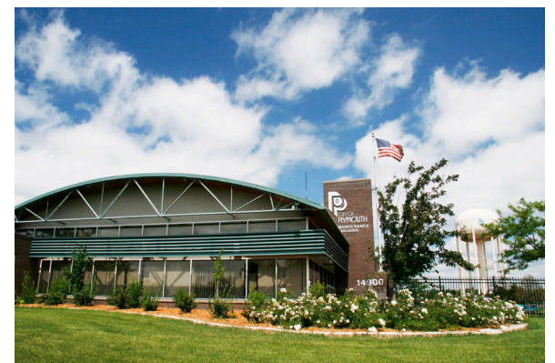
The Plymouth Maintenance Facility expansion project will add much-needed space to house the equipment, vehicles and staff needed to plow streets, maintain roads, and maintain the water and sanitary sewer system.
