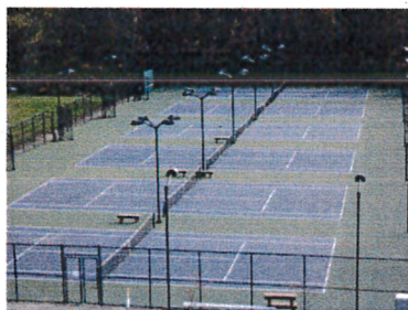
AGILENT TECHNOLOGY WILMINGTON, DE INSTALLED 2008
