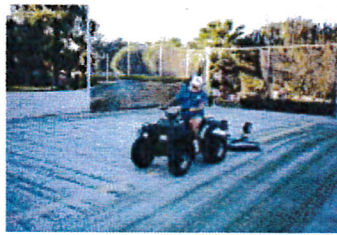
APPLY NATURAL SAND INFILL TO ACT AS BALLAST FOR SYSTEM
