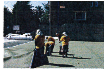
LAYING THE STRATUM LAYER A THERMALLY AND DIMENSIONALLY STABLE SYNTHETIC TURF
