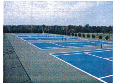
GETTYSBURG HS GETTYSBURG, PA INSTALLED 2009
