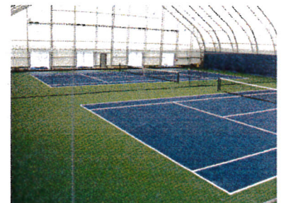
TEAM JAMIRI TENNIS PHILADELPHIA, PA INSTALLED 2006
