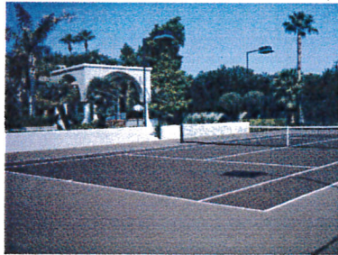
CAROLLO RESIDENCE PARADISE VALLEY, AZ INSTALLED 2000
