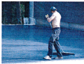
SQUEEGEE APPLY APPROVED FLEXIBLE BASE COAT OF ACR BINDER
