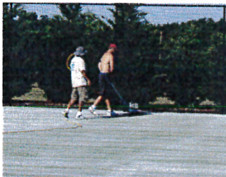
PREPARE STABILIZED STRATUM LAYER FOR THE FLEXIBLE COLOR FINISH
